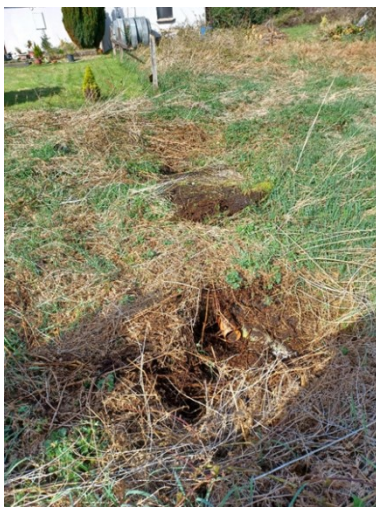
OUTFLOW PIPE FROM SEPTIC TANK DISCONNECTED FROM PERCOLATION AREA
