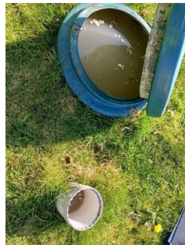
INADEQUATE PERCOLATION CAUSING EFFLUENT TO BACK UP IN SYSTEM
