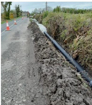
DRAINAGE WORKS ON THE R350 REGIONAL ROAD AT BENMORE TO IMPROVE ROAD SAFETY
